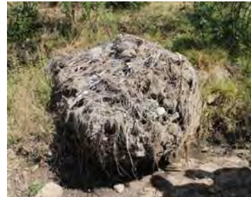
Gabion for gully
