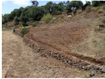
Stone bund and trench
